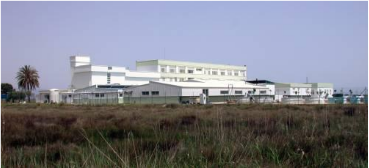
View of the 4 buildings (A-D) which compose installation IATS-EXP within the campus of the Instituto de Acuicultura Torre de la Sal.
