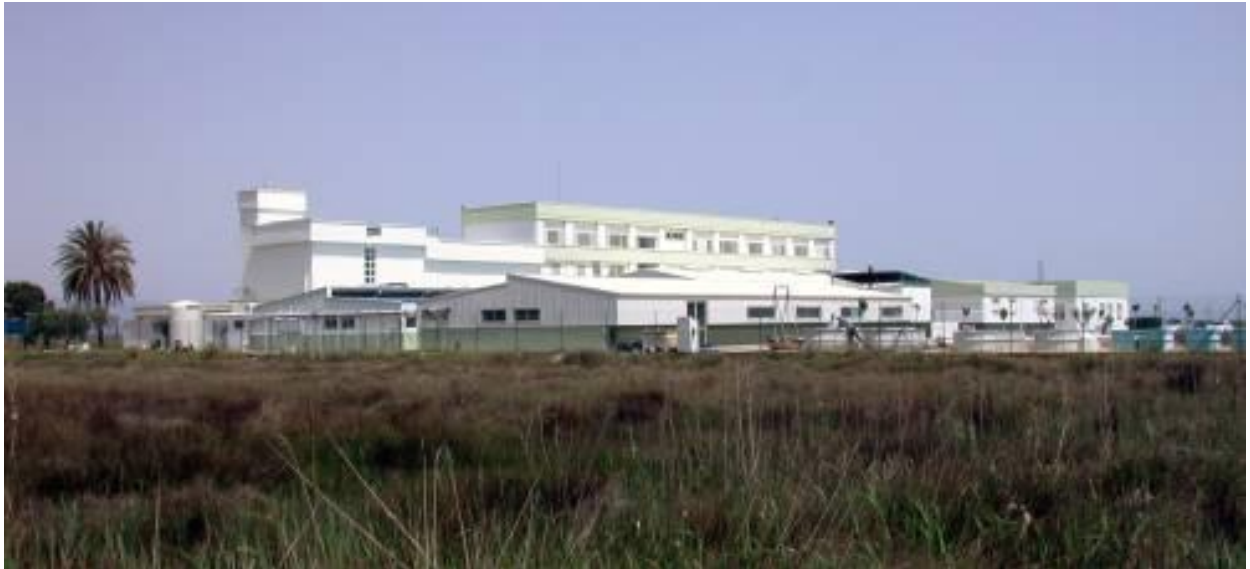
View of the 4 buildings (A-D) which compose installation IATS-EXP within the campus of the Instituto de Acuicultura Torre de la Sal.
