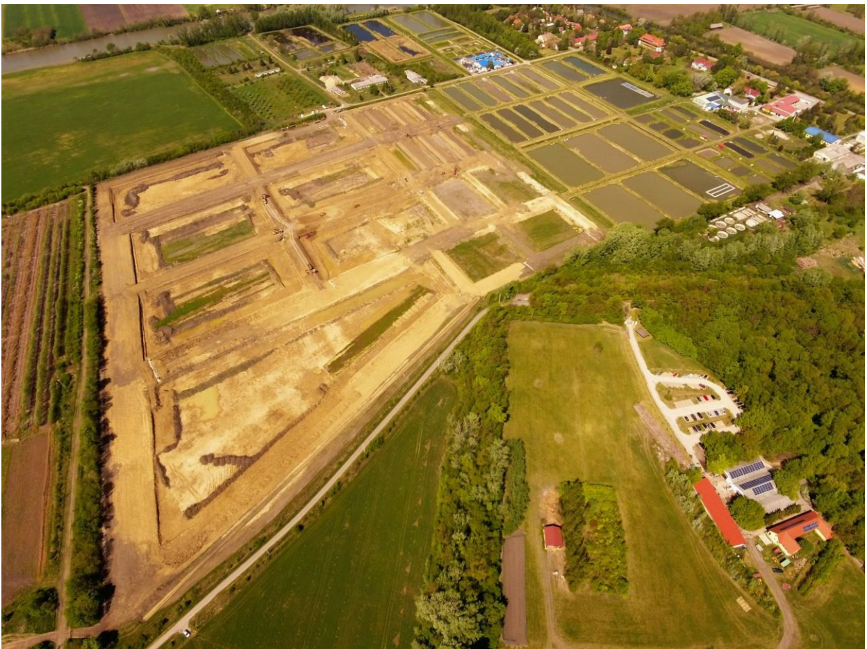
Fig. 1. HAKI OEPS installation.
